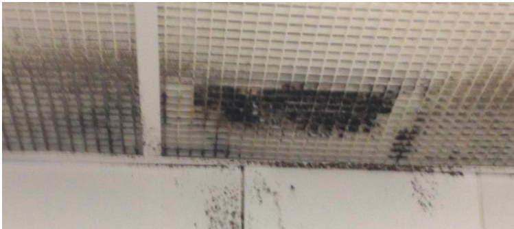
Figure 1. Visible mold on cold room ceiling grid and wall.
