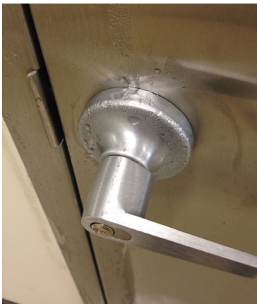
Figure 3. Visible condensation on cold room door handle.
